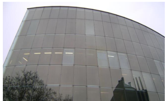
Figure 1. Bussiness Promotion Center, Duisburg, 1993. One of the earliest examples of simple double glazed façades. Arch.: Richard Rogers.
