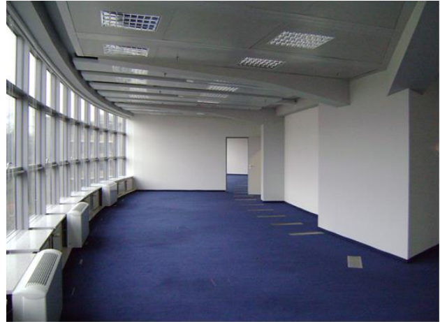
Figure 4. Hallenseestrasse Office Building. Interior office space; that remains unused because of the poor environmental performance of the building: on the left; the hvac set up in an attempt to fix this.
