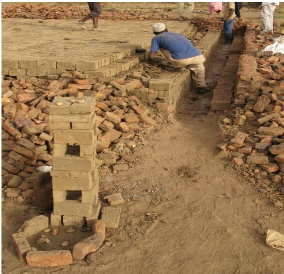
7. Loading of dried raw bricks in layers for burning
