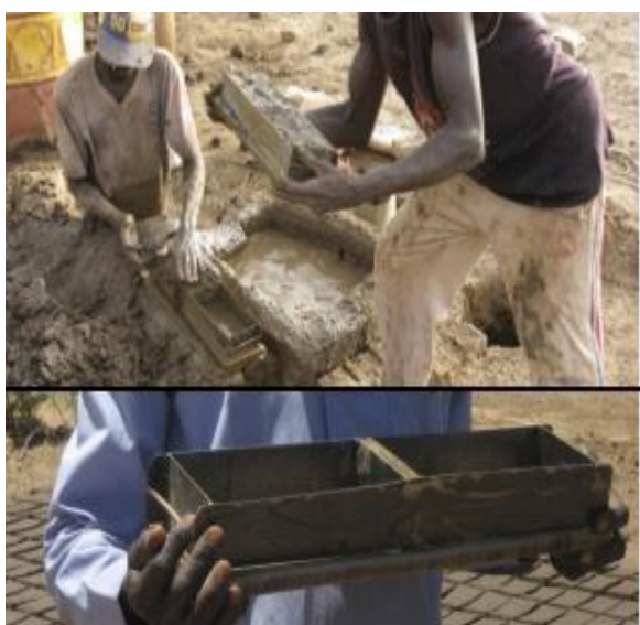
5. Forming of the mixture to bricks units using steel or wooden mould
