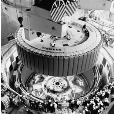
Figure 11: Hydroelectric plant Itaipu, Brazil, 1978; inserting the huge rotor into the stator; Siemens Corporate Archives
