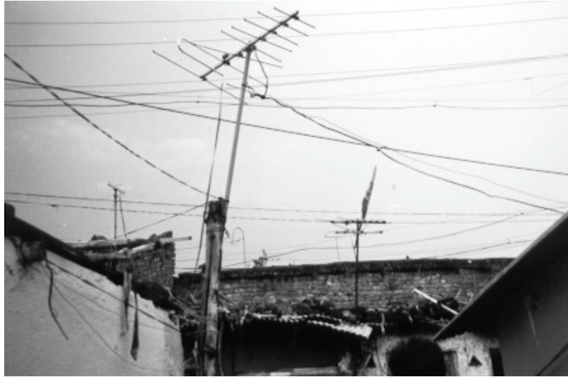
Figure 2.21 Illegal electric connection
