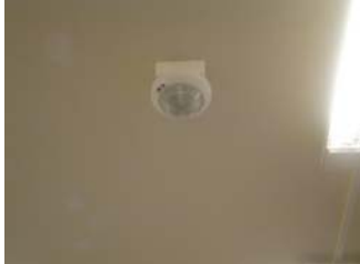
Figure 2.11b: Boox KNX/EIB Presence detector next to the lights.
