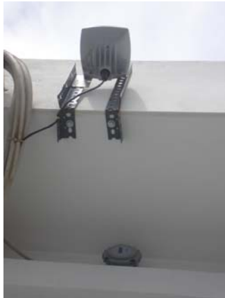
Figure 2.12b: Ambient temperature and solar radiation on a horizontal surface sensors.
