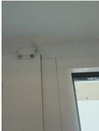
Figure 2.9b: Window reed contact.
