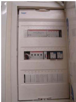
Figure 2.8b: KNX/EIB Boox Binary Input in the distribution board with the Power Supply, the Binary Output, etc.
