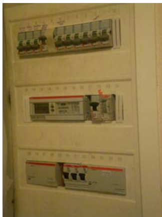
Figure 2.10b: KNX/EIB Boox Delta-Energy Meter with the Binary Output and Dimmer Actuator in the distribution board.
