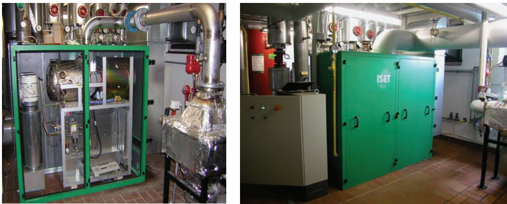
Figure 6-12 The microturbine under test at Eichhof (to the left is the system without the cabin doors and to the right the same system in the closed cabin)
