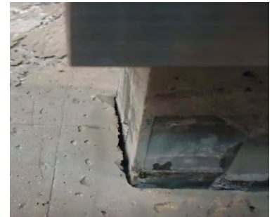
Fig. 9: Cracks after plastic hinges
