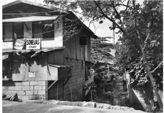
Figure 4e. An example of a non-engineered composite construction of masonry (first floor) and wood (second floor). The first story is partly used as a small neighborhood retail store.
