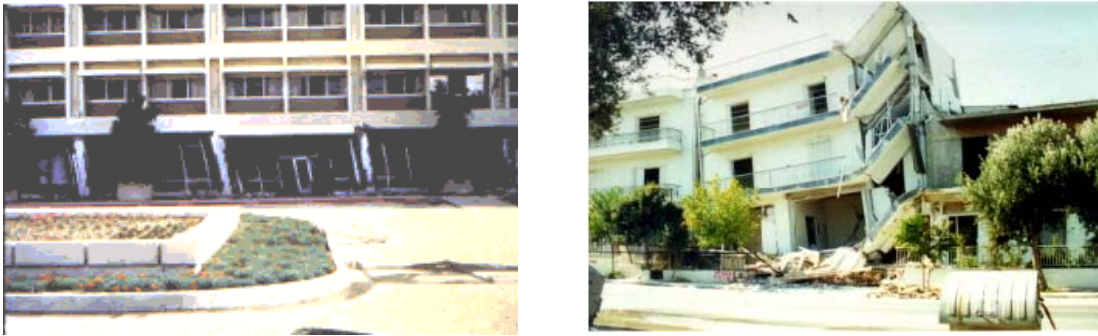
Figure 4v. Soft ground story collapse of Olive View Hospital in the 1971 San Fernando earthquake (left) and (pilotis) collapse of a poorly constructed four-story RC apartment in the 1999 Athens earthquake (right). Pounding could have occurred as evidenced by heavy damage on the right side of the taller building. (Sources: BSSC, 1995b; Dimitriu, 2000.)
