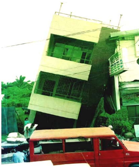
Figure 1b. The foundation of this building in Dagupan City failed due to liquefaction. (Source: PHIVOLCS website.)
