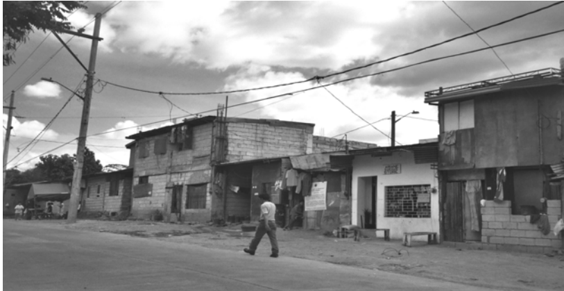
Figure 4f. This photo shows the diversity in the types of single-family residential houses in Marikina City. This row of houses is fronting a major thoroughfare in a traditional, non-subdivision neighborhood. Substandard structures such as one-story non-engineered unreinforced masonry (extreme left) and masonry-cum-wood houses (extreme right) and non-engineered two-story RC houses are commonly seen in similar quarters around the city. Take note again the use of residential space for petty commercial activity (building second from right).
