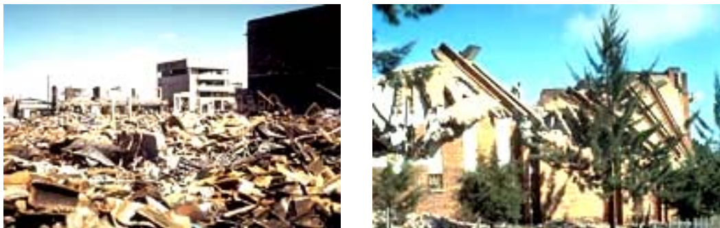
Figure 4t. Downtown Managua City, Nicaragua after the 1972 Managua earthquake (left). The total collapse of URM and adobe buildings left 5000 people dead because of falling masonry walls and roofs supported by these walls. Complete collapse of an unreinforced brick masonry church during the 1976 Guatemala Earthquake (right). (Source: Bertero, 1985)
