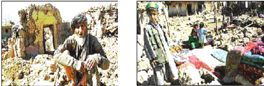
Figure 4u. Traditional mud brick houses in Afghanistan easily collapsed and left thousands homeless as a result of the 7.4 magnitude earthquake in 2002.
