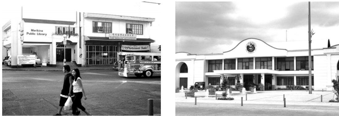
Figure 4n. Institutional buildings such as the Marikina Public Library (left) and the City Hall (right) are located in the traditional commercial district.
