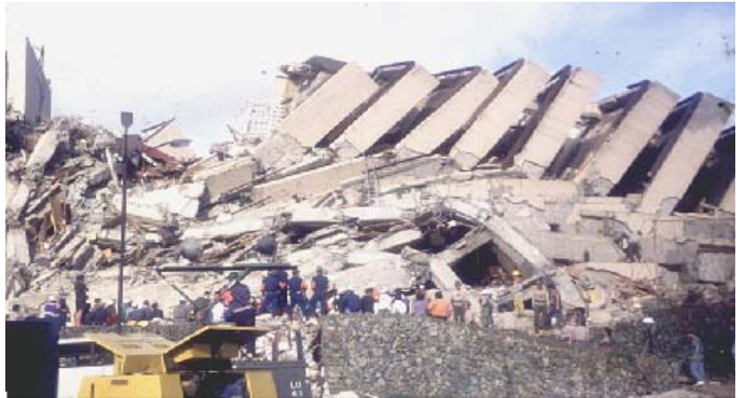
Figure 1a. Five-star Hyatt Terraces Hotel in Baguio City collapsed due to strong ground shaking. (Source: PHIVOLCS website.)
