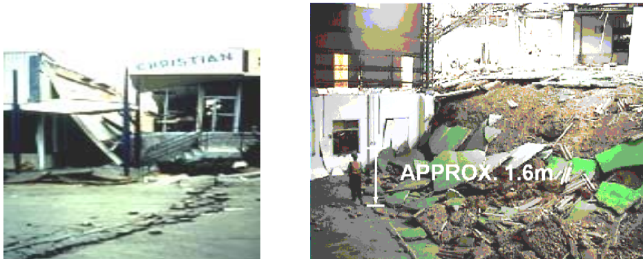
Figure 4y. Damaged to a building in Sylmar during the 1971 San Fernando earthquake (left) and vertically displaced structures along the fault caused by the 1999 Chichi, Taiwan earthquake (right). (Sources: Bertero, 1985; O'Rourke, 1999.)
