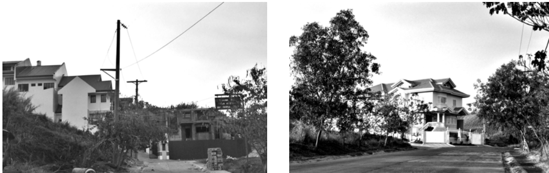
Figure 4i. A two-story reinforced concrete house is under construction across the street from a row of townhouses (left) and an example of a two-story residence in a low-density residential area.
