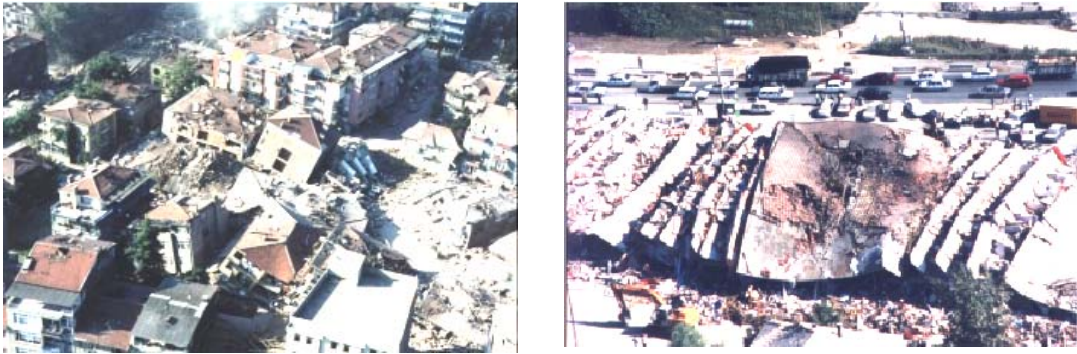
Figure 4r. Poorly built medium-rise RC apartment blocks pancaked during the August 1999 Duzce (left) and November 1999 Kocaeli earthquakes (17,000 people killed) (right) in Turkey. (Source: Erdik, 2000.)
