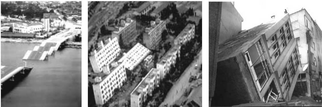
Figure 4x. Effects of liquefaction show in the collapse of the Showa Bridge by falling off its piers (left) and in the tilting of apartment buildings (center) in Japan after the M=7.5 1964 Niigata earthquake and in Adapazari after the 1999 Kocaeli earthquake in Turkey. (Sources: Bertero, 1985; Erdik, 2000.)
