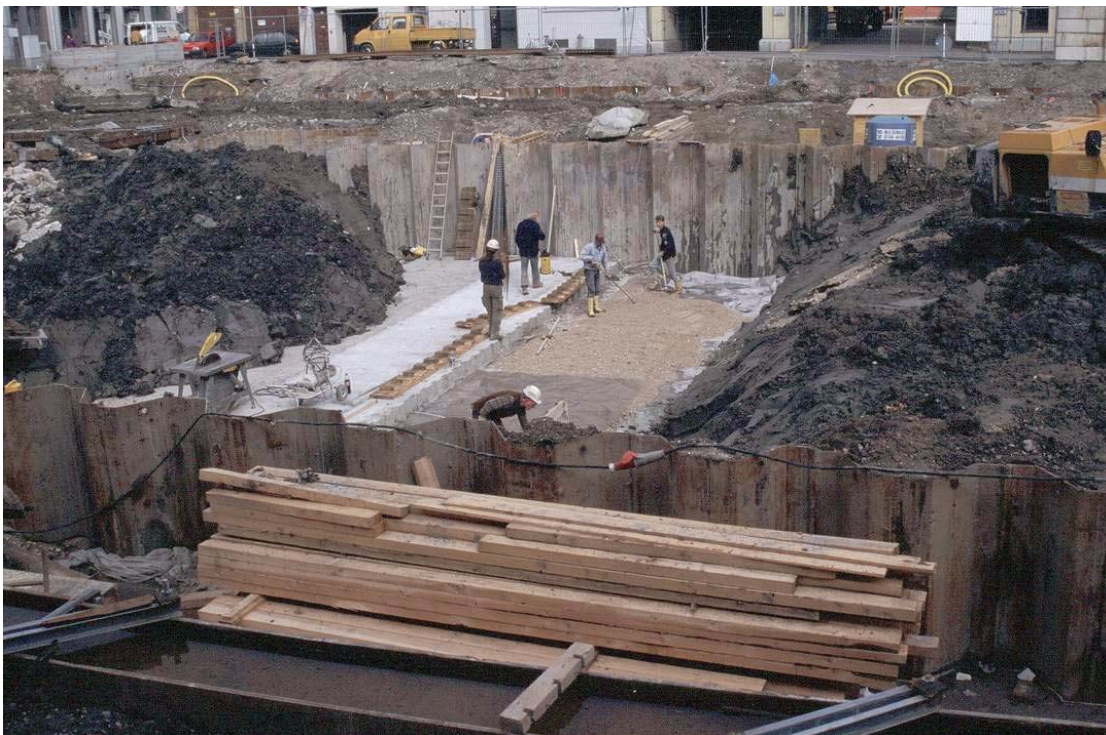
Figure 8.5: Excavation and placement of the bottom slab in slices [Photo: Kempfert]
